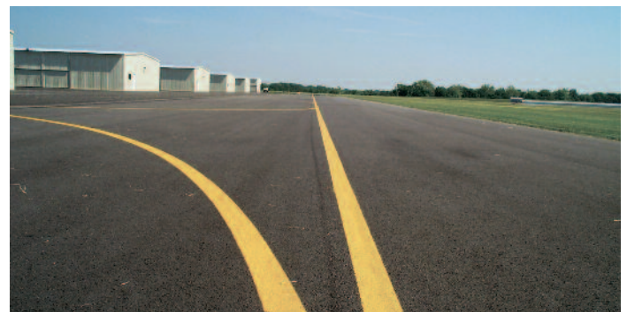
Taxiway markings are yellow. The centerline is a single yellow line, and the taxiway edge is marked by a double yellow line. Dashed edge markings allow the aircraft to cross to the adjoining apron.
