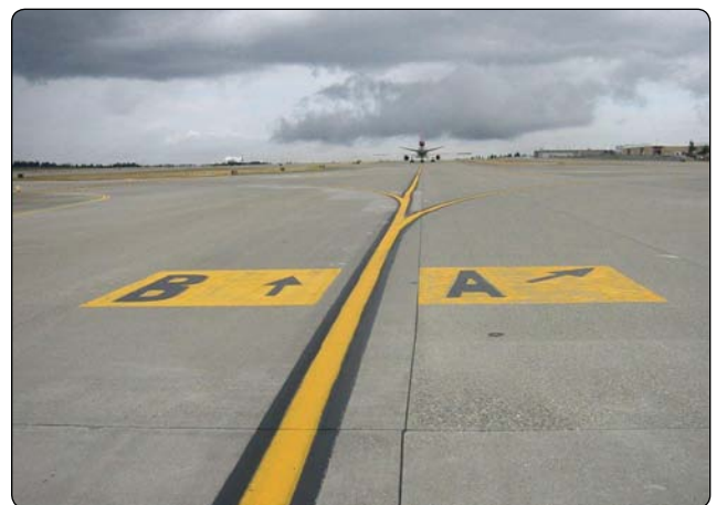
Figure 1-32. Surface painted taxiway direction signs.
