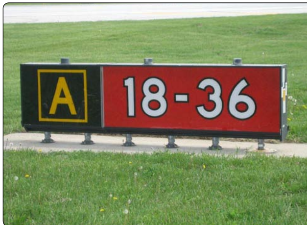
Figure 1-20. Runway holding position sign at a location other than the takeoff end of Runway 18-36 with collocated Taxiway Alpha location sign.
