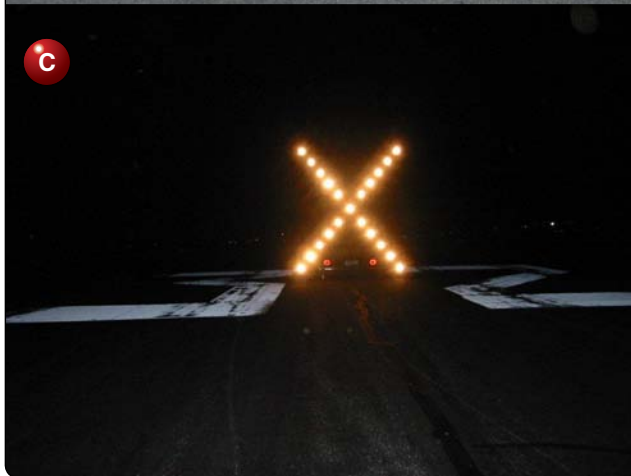
Figure 1-39. (A) Yellow “X” placed on surface of temporarily closed runways. (B) Lighted “X” placed on temporarily closed runways. (C) Lighted “X” at night showing a temporarily closed runway.
