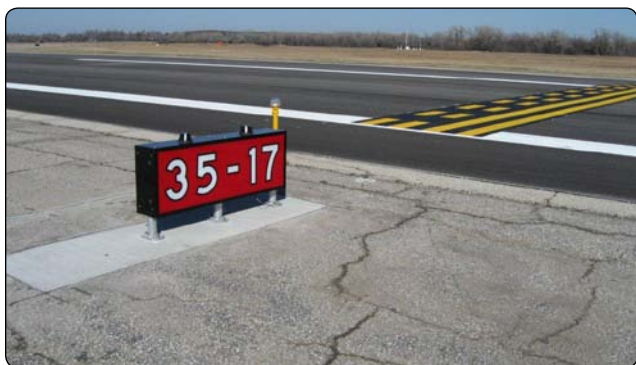
Figure 1-28. Runway holding position sign and marking for LAHSO.
